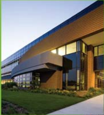
RFAB, located in Richardson, Texas, is the world's first LEED-certified semiconductor manufacturing facility.
