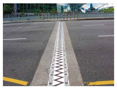
Figure 1. Expansion Joint on a Bridge in Order to Prevent Cracking
