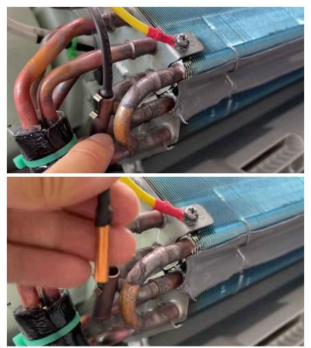
Figure 1-2. Position of the Temperature Sensor for Evaporator Coil
