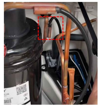
Figure 1-5. Compressor Discharge Temperature Sensor Installation
