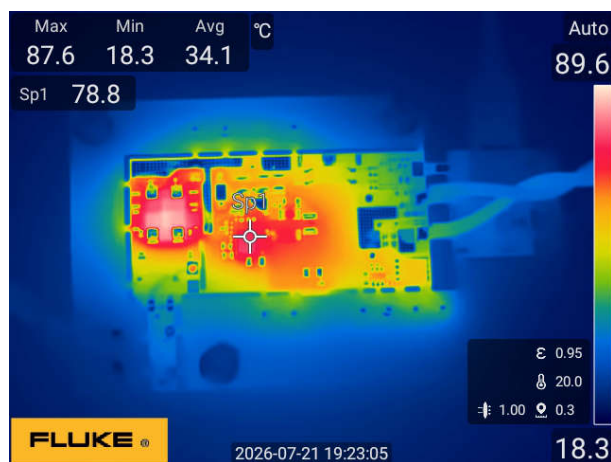
Figure 3-81. Bottom Side at 115Vac-to-20V/3.25A
