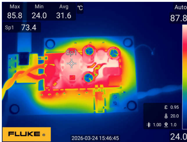
Figure 3-78. Top Side at 90Vac-to-20V/3.25A
